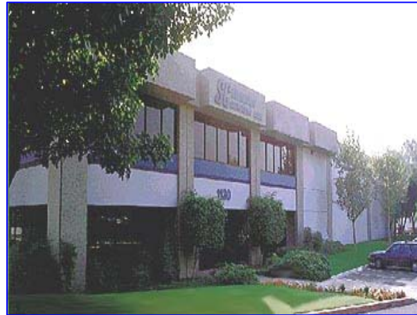
In a 65,000 square foot facility, SC Hydraulic is capable of setting the industry's highest standards while maintaining the best delivery times
